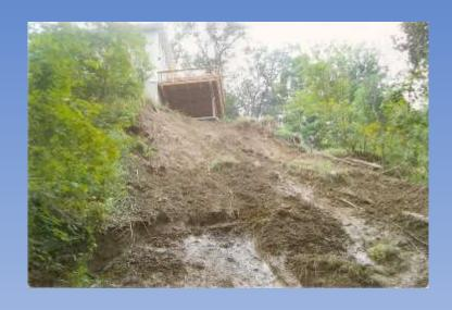
SES completed work to stop further damage to slope by tying residential downspouts to drain line down to creek.
